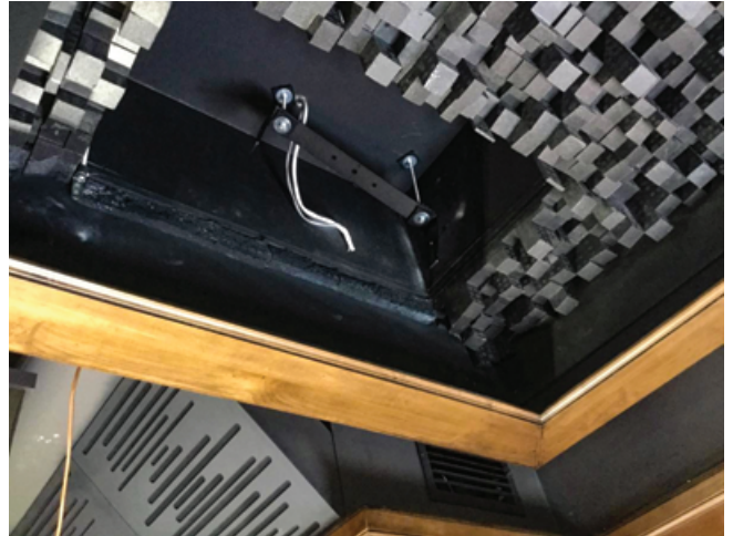
Special bracketry aimed the front, center and back tops aimed in TRINNOV RECOMMENDED crossfiring aimings.
