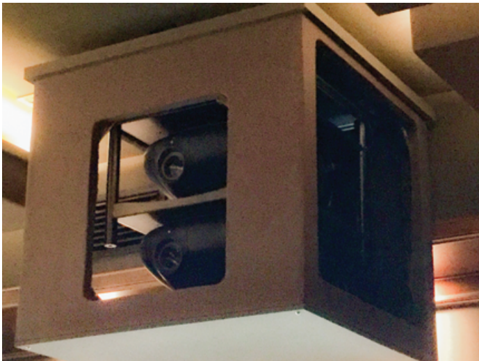
Bespoke ventilated projector stack hushbox.
